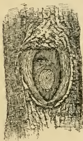
104. Plugging a cavity.
